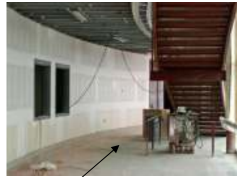
Looking south to north on the curved wall.
