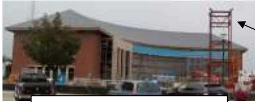
Construction Aug above, Sept. below
