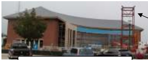
Construction Aug above, Sept. below
