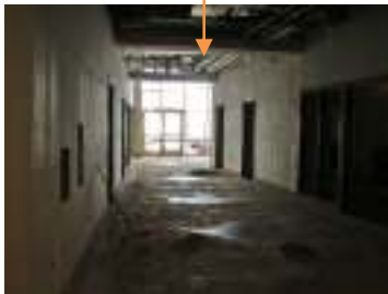
Terrazzo floor poured not sanded looking from west to east.
