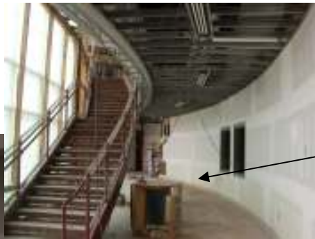
Terrazzo floor poured not sanded looking from west to east.
